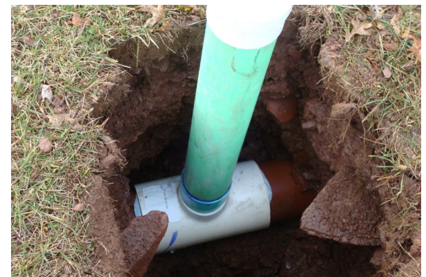
Cleanout Installation of lateral for lining
