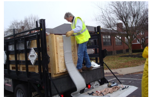
Cure In Place Lining of Main Sewer Pipe
